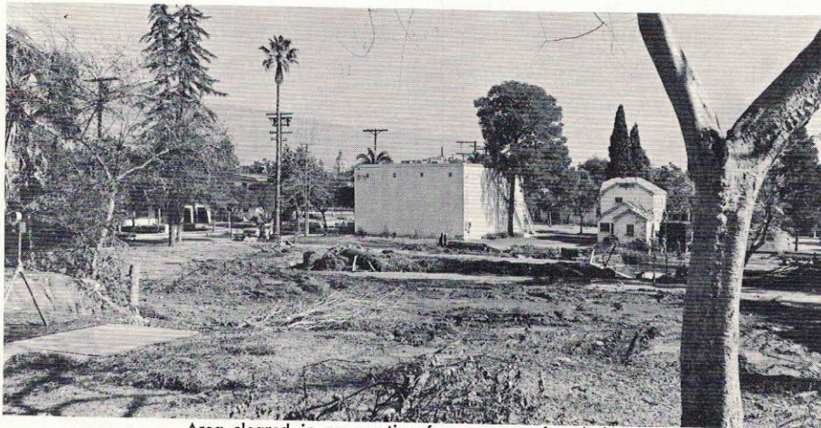
Area cleared in preparation for new gym foundation.
